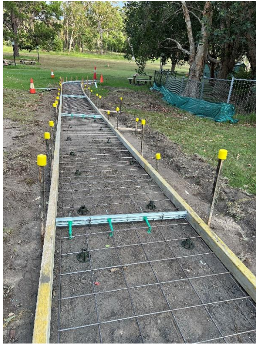
Fig. 6.7: Prepared site for footpath application.
