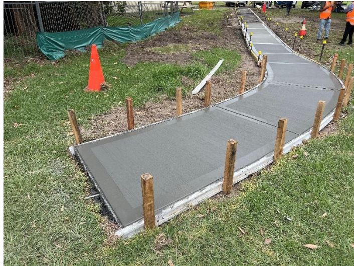
Fig. 6.11: Footpath after surface finish.
