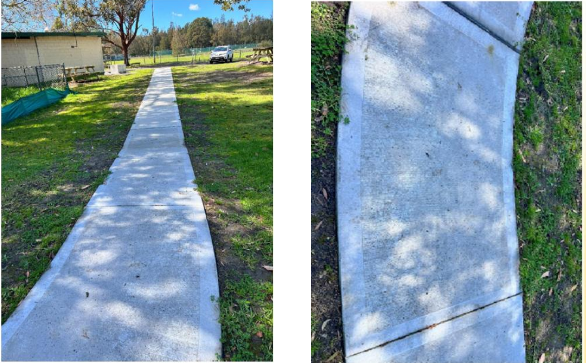
Fig. 6.20: FBA concrete pavement.
