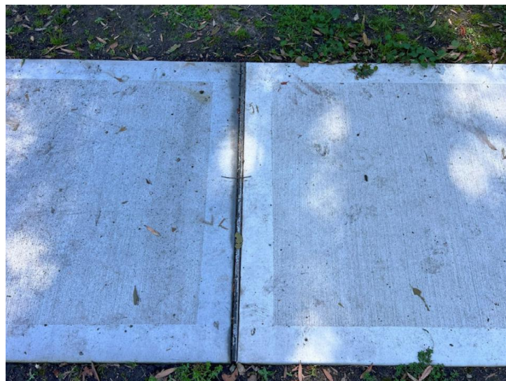
Fig. 6.19: FBA concrete (Left) and Control concrete (Right).
