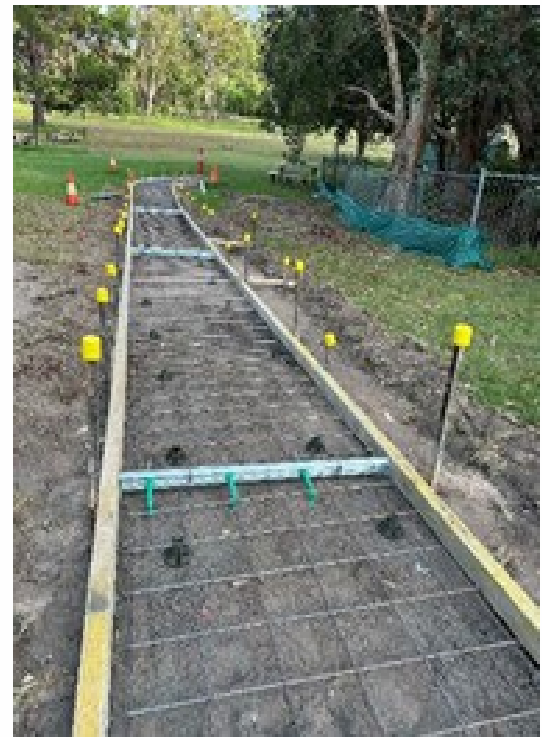
Figure 13: The trial footpaths construction
