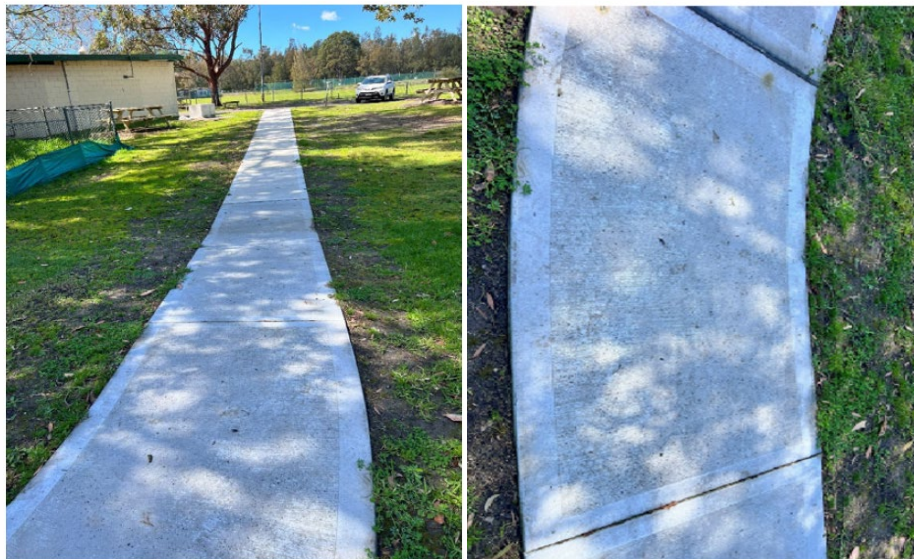
Figure 17: FBA concrete pavement: Surface appearance after two months
